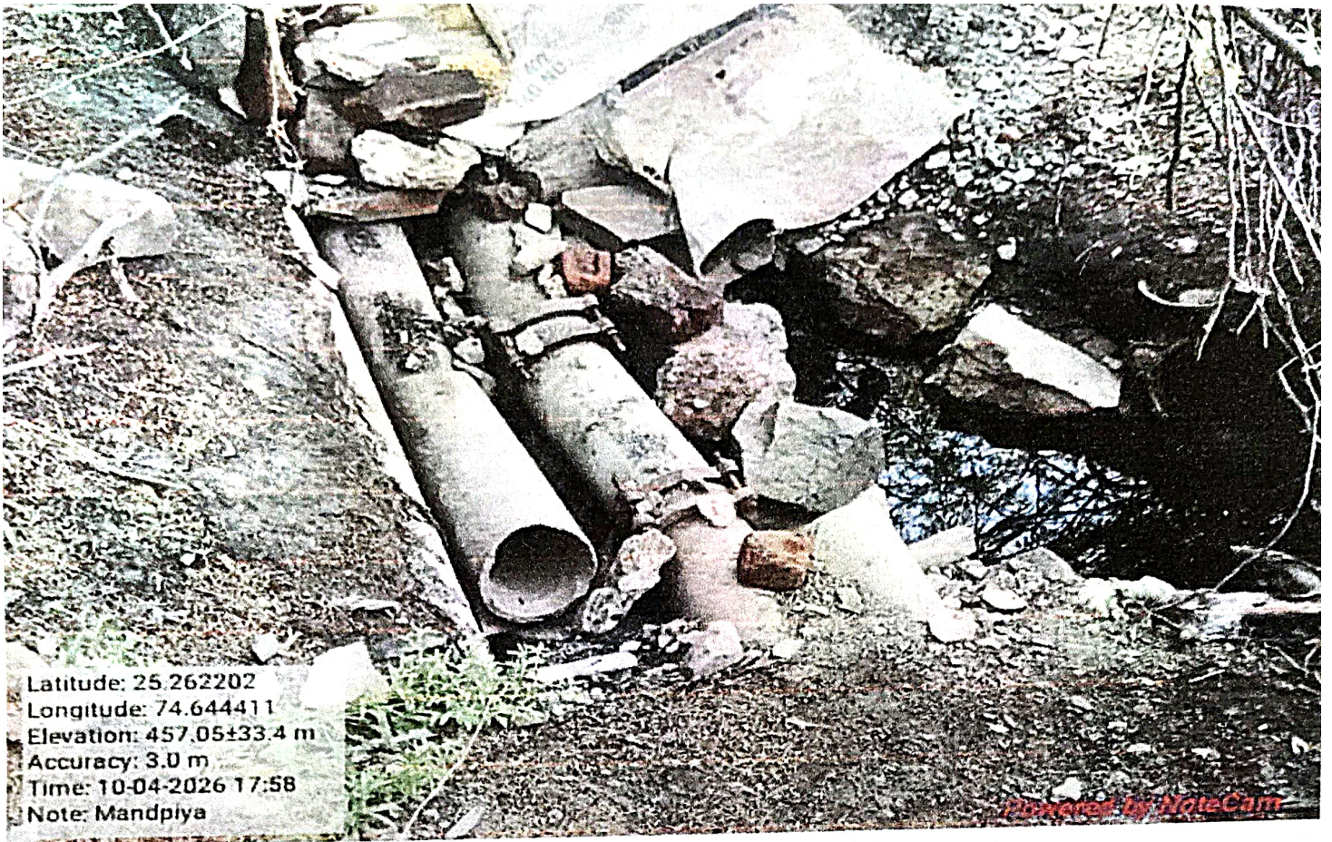
Figure 3. Nut Bolt arrangement attached with Pipe line at Mandapiya unikt of M/s Anant Syntex Ltd
